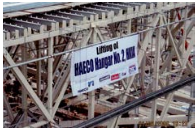
Project: Haeco Aircraft Maintenance Hangar No. 2 Hong Kong
